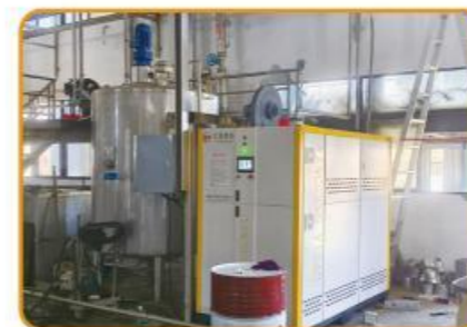
柴油模温机供热交换器 Diesel model temperature machine heating exchanger
