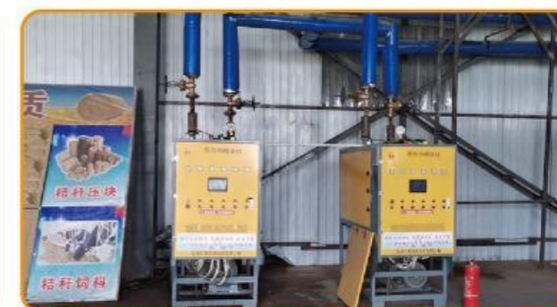
辽宁化工厂 Liaoning chemical plant
